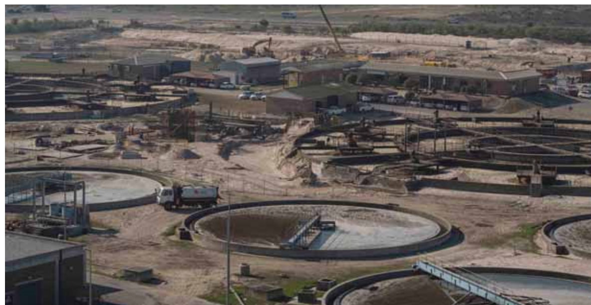
Making the most of water: The City's biggest capital project in the east of the metro is the work at the Zandvliet wastewater treatment works. This R445 million project will provide increased capacity and extensive water reuse, reducing demand on the dams.
