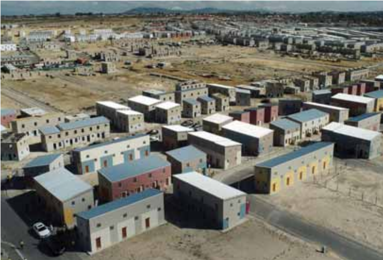
Going up. The 4 820 unit Blue Downs housing project is a quarter complete.
